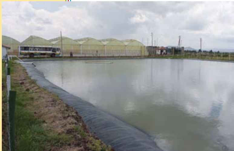
Rain water is collected in an enormous reservoir.
